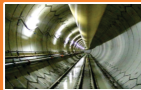
Kishanganga Hydroelectric Power Project - HCC
