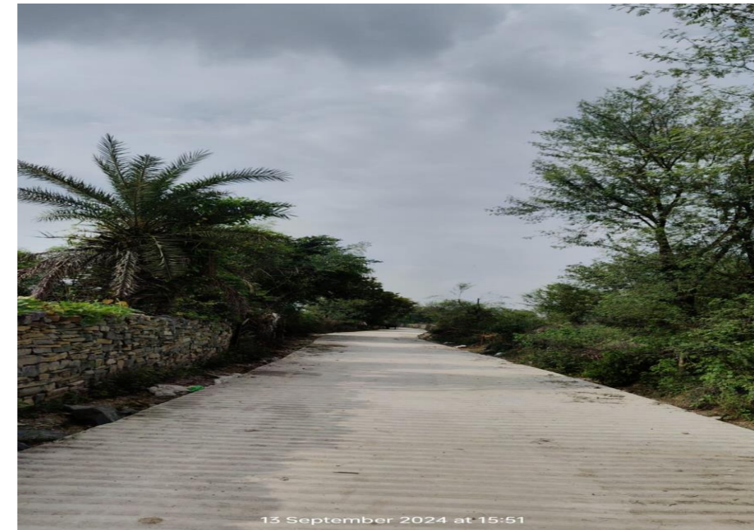
Construction of CC Road in Mangrol
