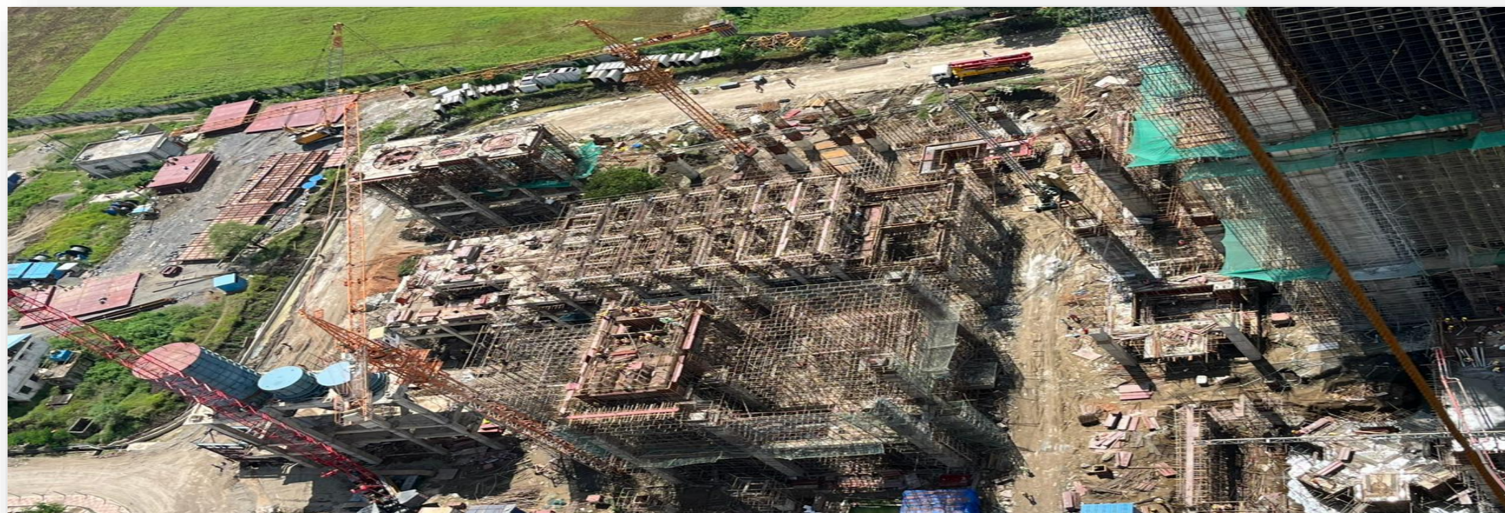
Raw Material Section –Panna Line-II
