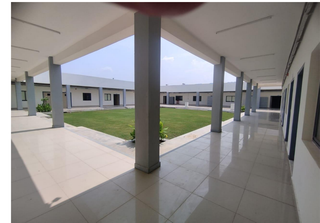
Construction of ITI at Panna
