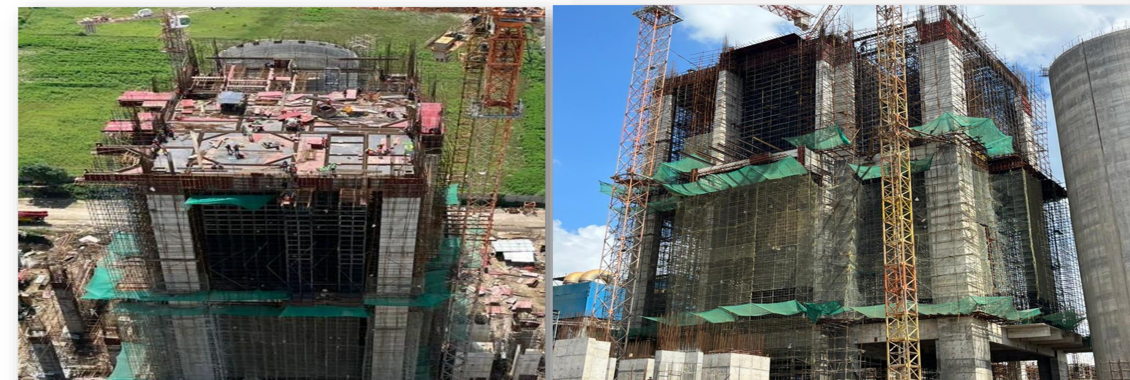
Preheater Building-Panna Line-II
