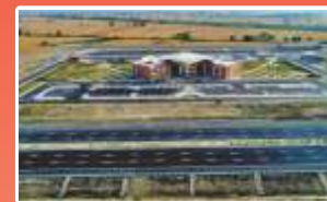
Agra Lucknow Expressway - AFCONS
