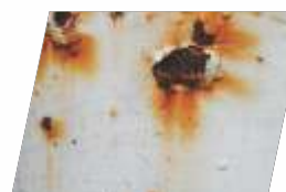
Corrosion of Steel
