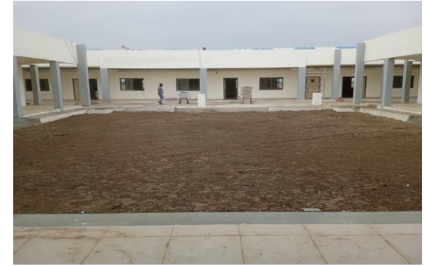
Construction of ITI at Panna
