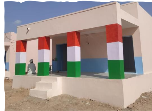
Renovation of Primary School in Gotan
