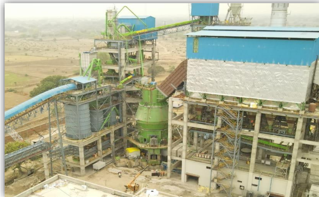
Hopper & Cement Mill
