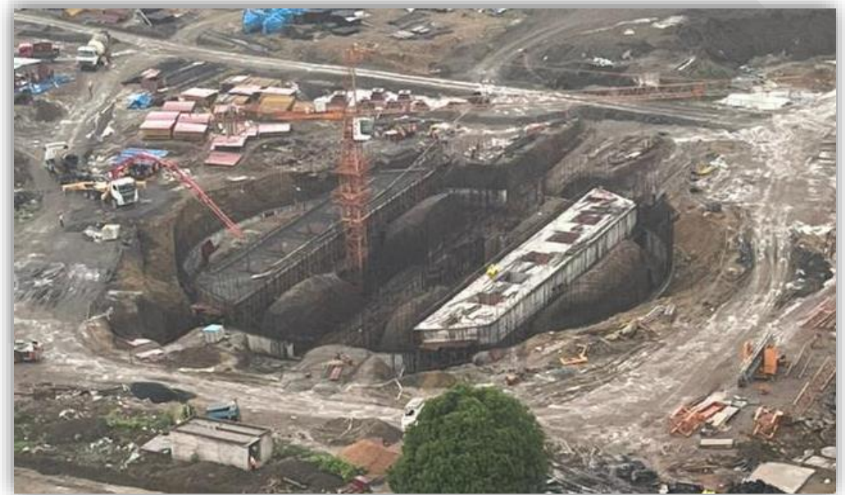
Clinker Silo Slab Casting
