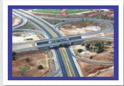
Eastern Peripheral Expressway
