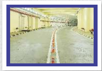
Atal Tunnel, Himachal Pradesh
