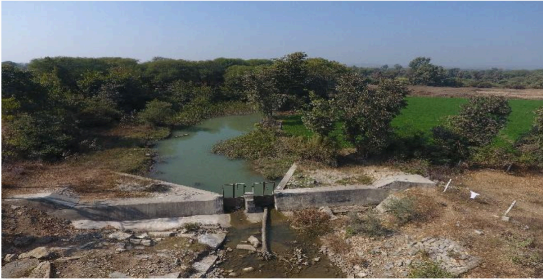
constructed an Anicut at Maliyakhaera village
