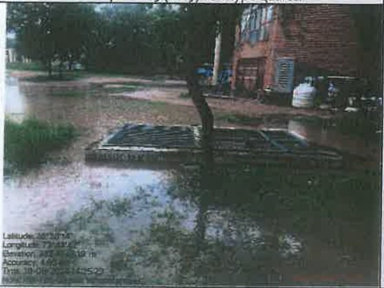
RWHP pit no. 09 at School Canteen
