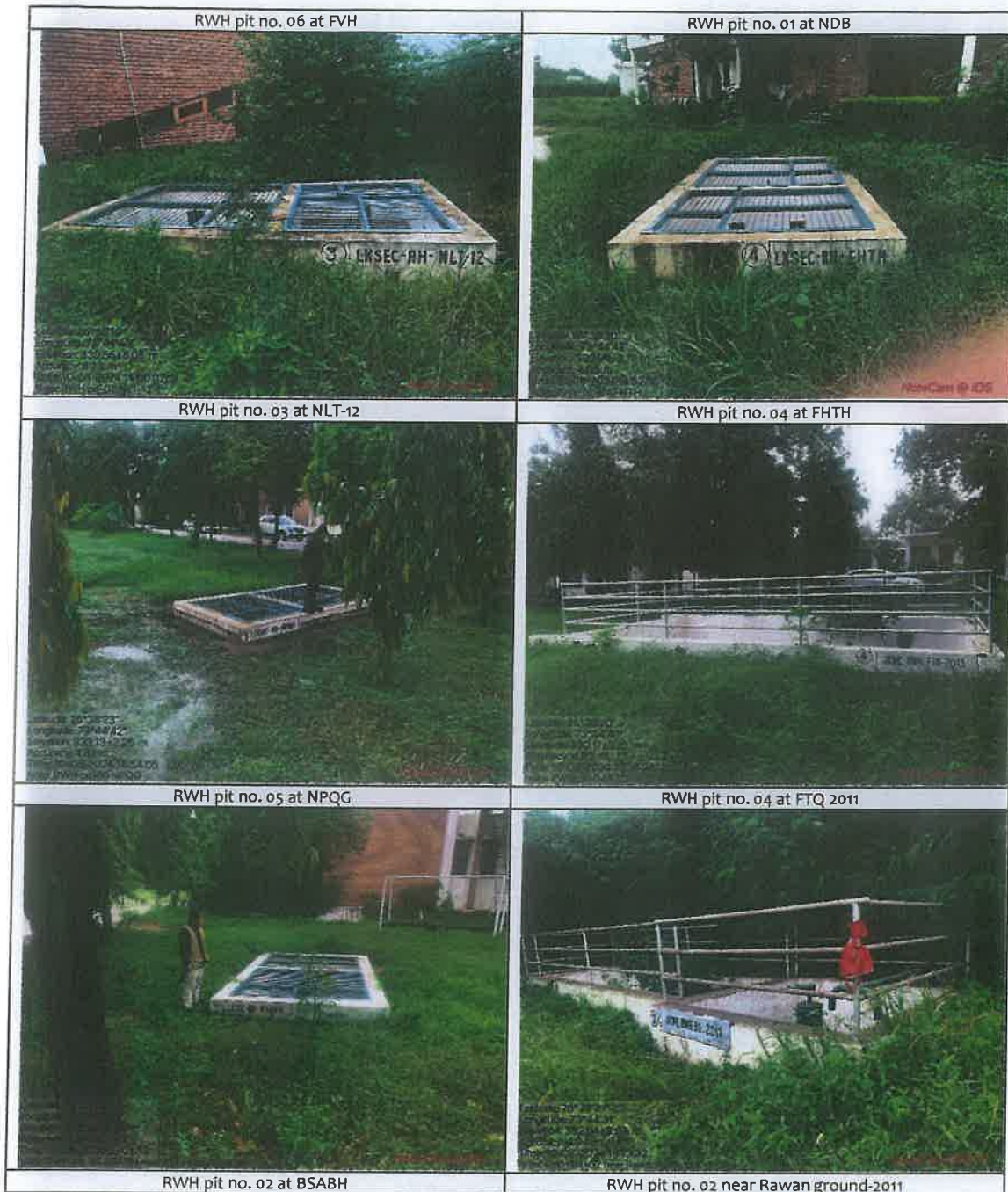
Figure 16: Thirty existing RWHP pits within JK White Cement Plant.
