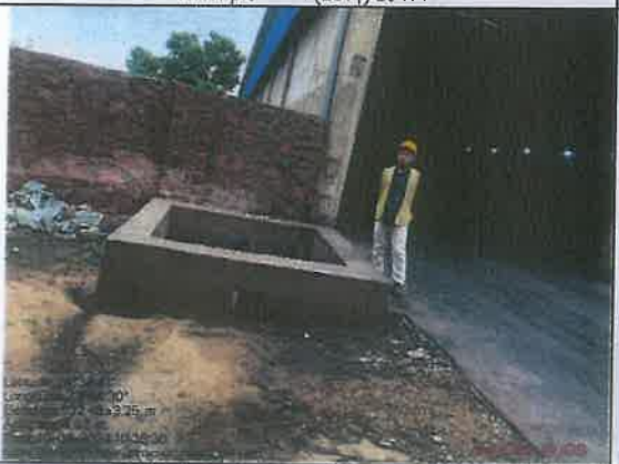
RWHP pit new (unnamed) near Coal Yard
