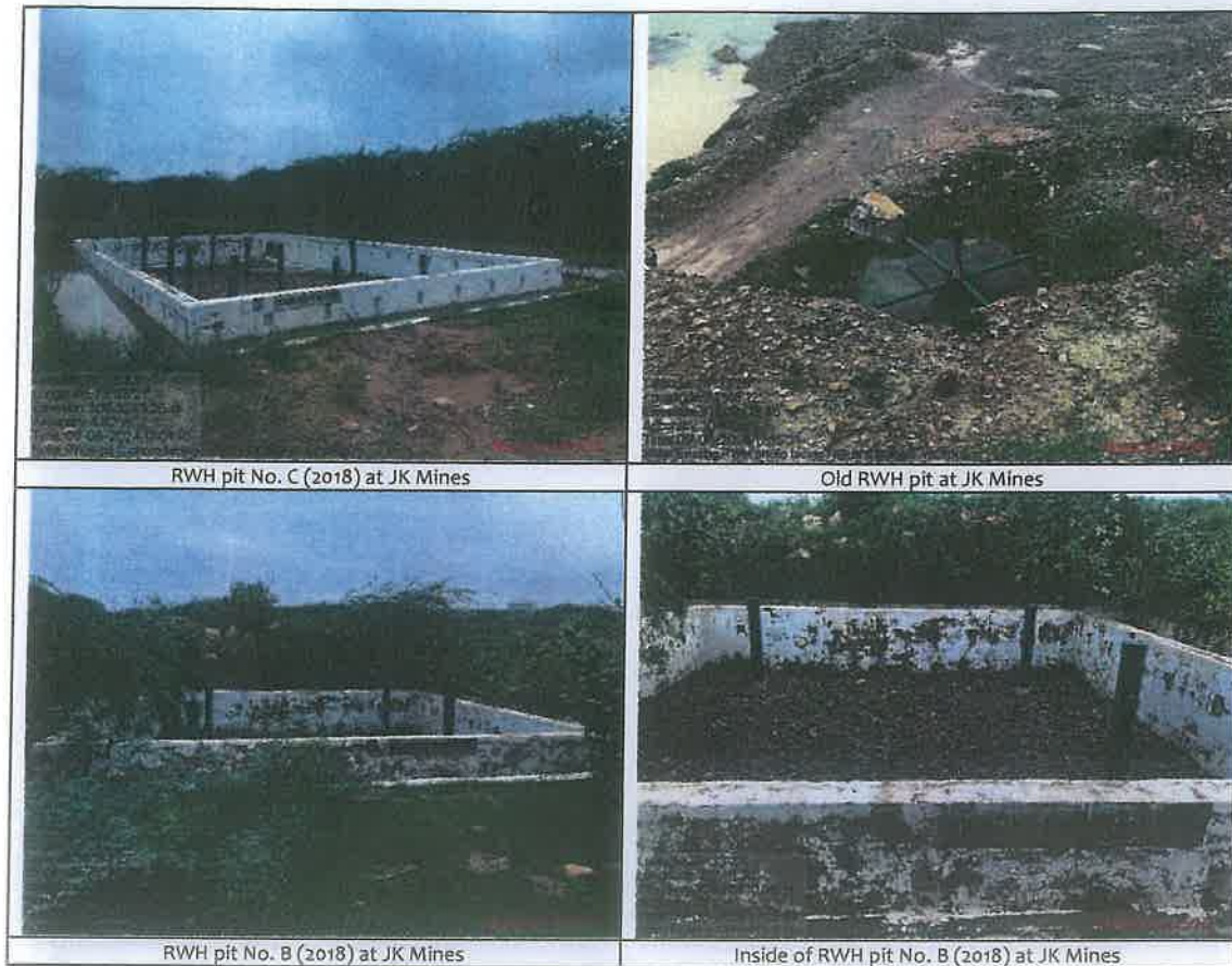
Figure 18: Three RWH pits at the operating mine site
