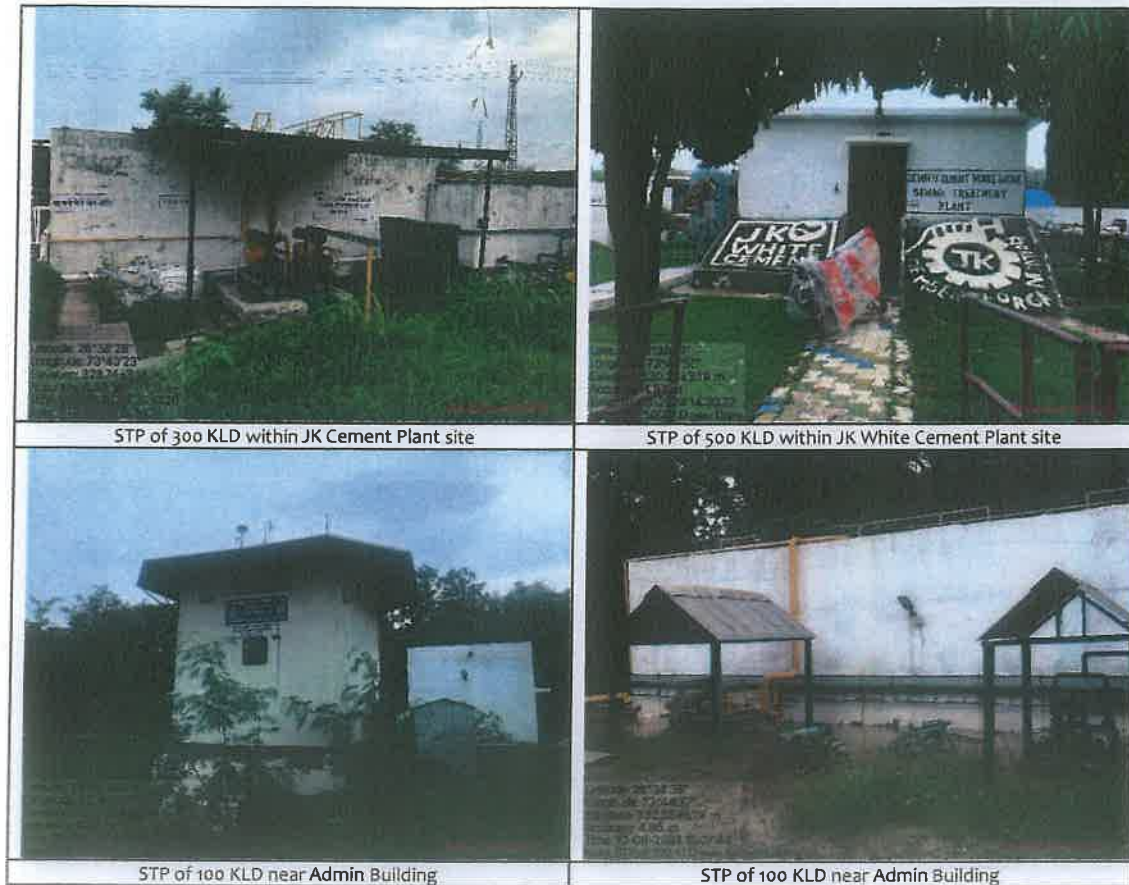
Figure 19: Three Existing STPs at JK Cement Plant.
