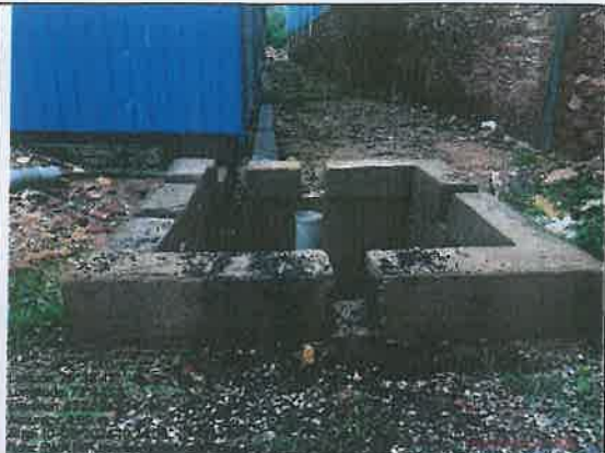
RWHP pit new (unnamed) near Coal Yard
