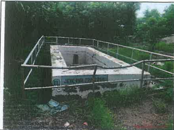
RWHP pit no. 11 (2014) at TPP
