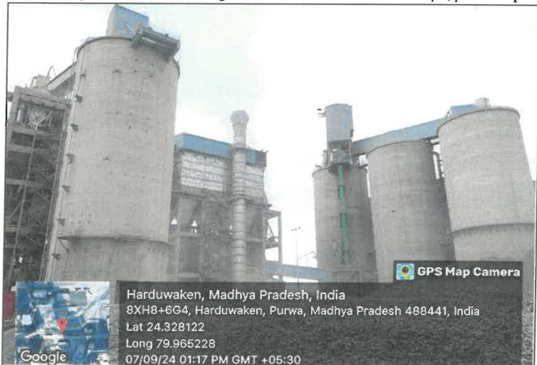
Picture 3- Flyash & Cement Silos
