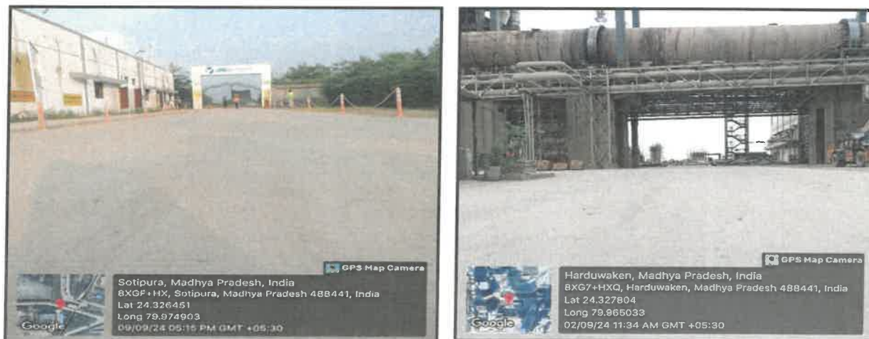
Picture 4- Paved roads and Paved floor
