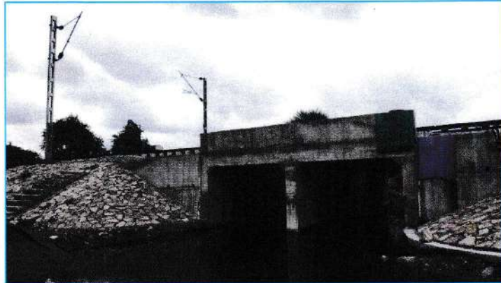
Plate 5.4. View of the underpass for drainage below the new railway line
