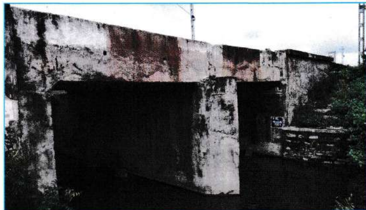
Plate 5.5. View of the underpass for drainage below the old railway line
