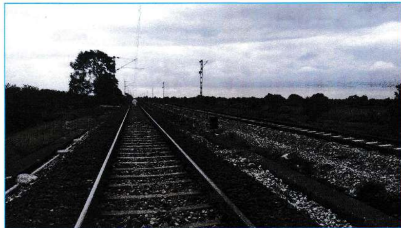
Plate 5.2. View of the Railway Line passing near the ML in the eastern side
