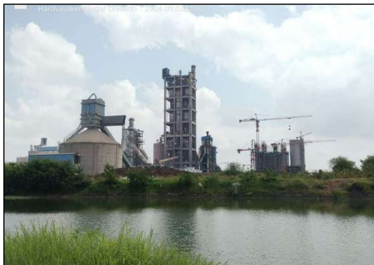
Rain water harvesting pond (30000m3 capacity)
