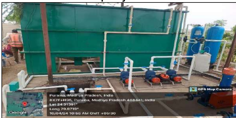
STP With Capacity 25 KLD
