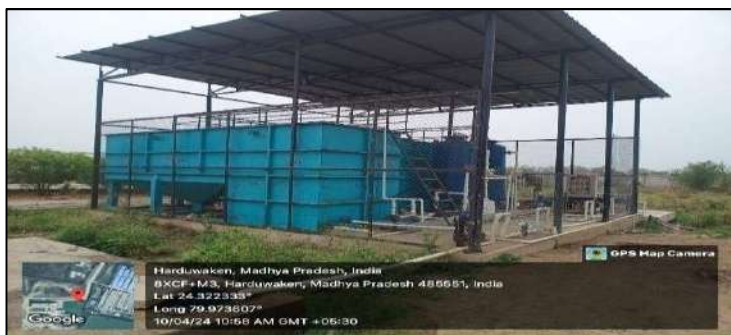
STP With Capacity 25 KLD
