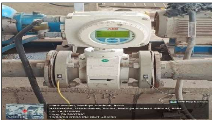
WHRS meter/DM inlet
