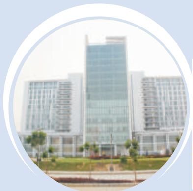
Vedanta Hospital (Medicity Project), Gurgaon
