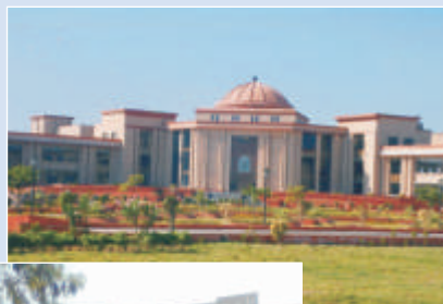
High Court, Bilaspur, Chattisgarh
