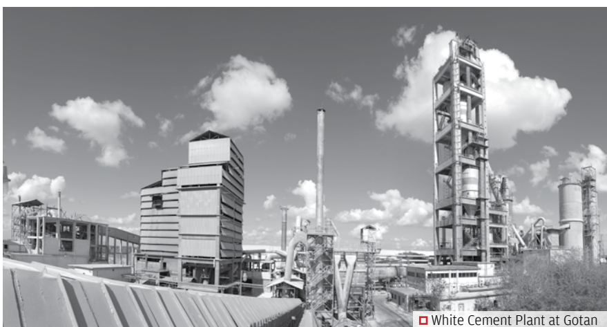
White Cement Plant at Gotan
