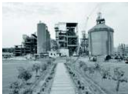
➤ Jharli plant view
